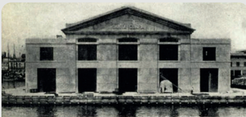
Below Right: PORT OF BUENAVENTURA, Republic of Colombia, S.A., showing reinforced concrete bulkhead 2376' long—four warehouses 150' x 292'—and newly made land comprising 47.6 acres. Depth of water alongside 32.8 at mean low tide—3412 PRECAST CONCRETE PILES ranging from 35 to 71' in length—work done for Colombian Government.
